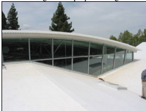
Figure 6.2: Example of a cool roof (fypower.org).
